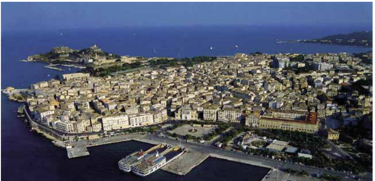
Fig. 4 -The city of Corfu today. Source: Google Earth.
