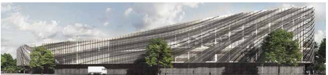
Fig. 22 - The bioclimatic design of the building resulted to the Natural cooling, passive heating and renewable energy production. Source: authors.
