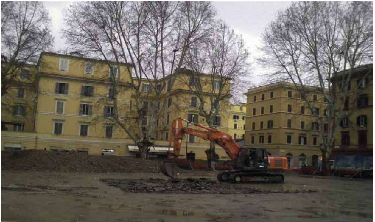
Fig. 1 - Piazza Testaccio: Regeneration works in progress.
