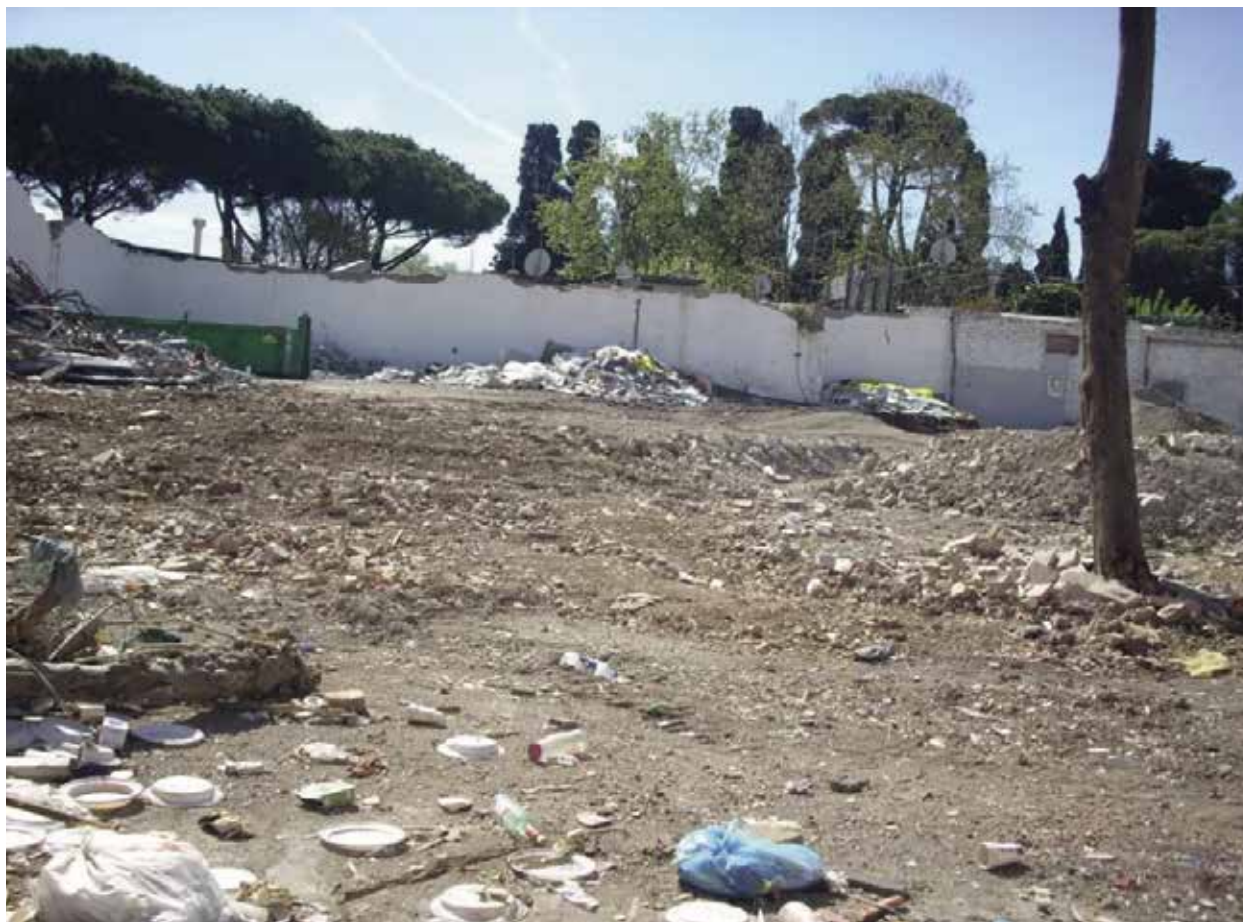
Fig. 5 - The demolition of an illegal settlement in Borghetto Caselli.
