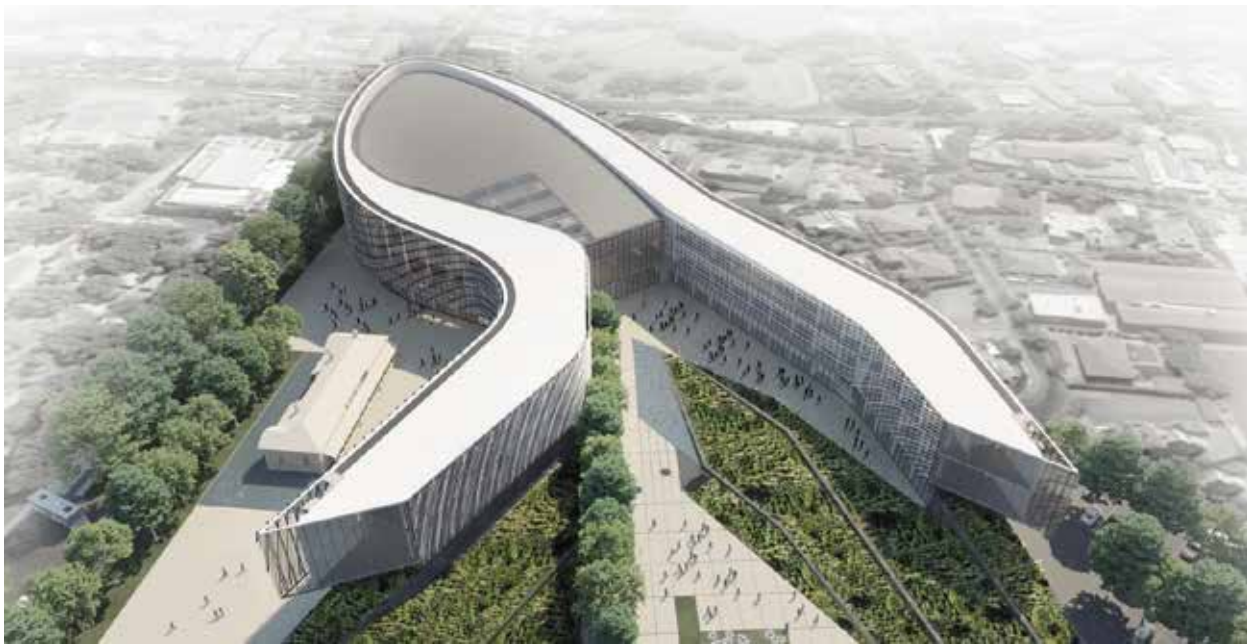
Fig. 23 - The Roof integrated photovoltaic panels, high performing batteries, widely sun shaded facades, LEED strategies and proper planting design result to the energy saving and improvement of the cooling. Source: authors.
