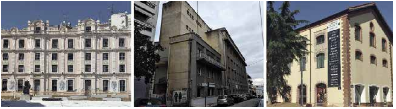
Fig. 3 - Municipal Tobacco Warehouse | National Tobacco Organization | Regie shopping mall (Images by the authors).
