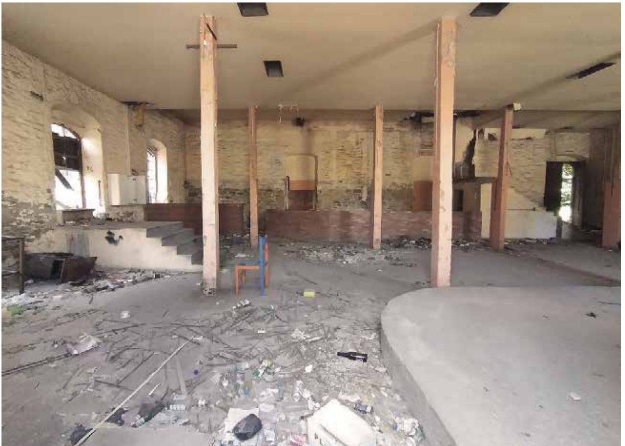
Fig. 4 - Interior hall of an abandoned warehouse (Image by the authors).
