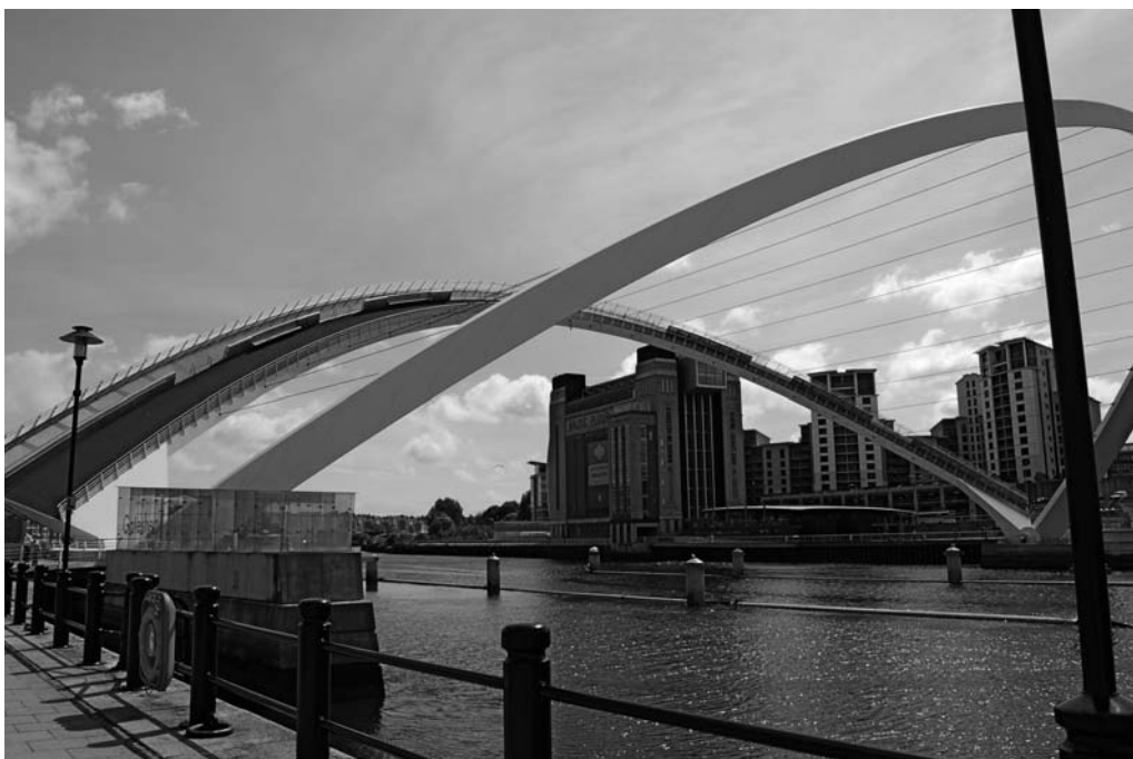
Fig. 2 - Il Millennium Bridge in movimento, davanti al Baltic Centre for Contemporary Arts
